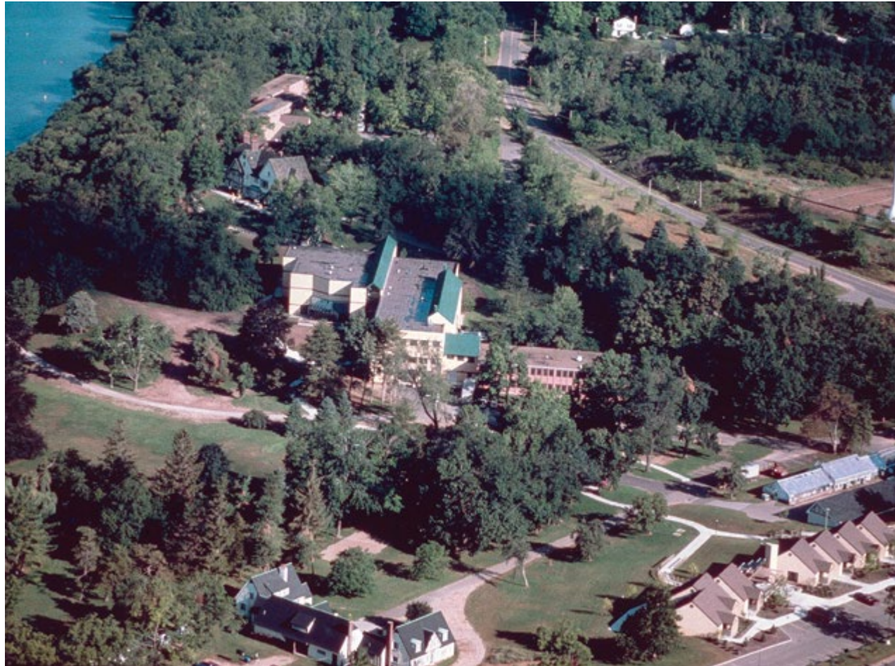
Aerial view of the KBS academic complex on Gull Lake in the early 1980s, showing the Academic-Stack research and education center and historical buildings built as part of W.K. Kellogg's summer home, Eagle Heights, in the 1920s.
